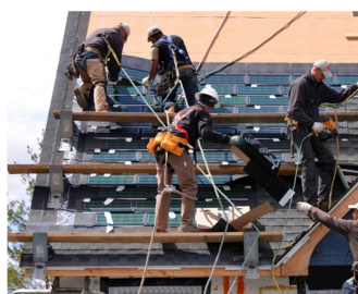
Installation of solar roof shingles at the Shore Road project.
